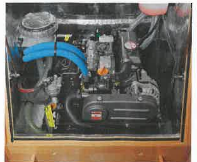
Engine access is okay but access to oil filters and the impeller cover is limited
