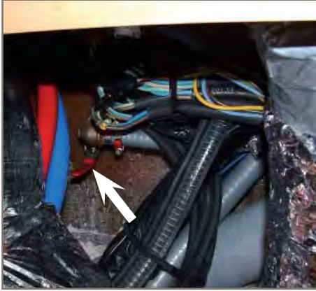
OUTLET VALVE WASHING MACHINE
