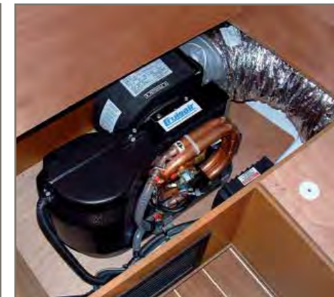
AIR CONDITIONING UNIT
