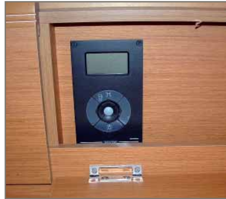
CONTROL OF THE TRANSFER PUMP
