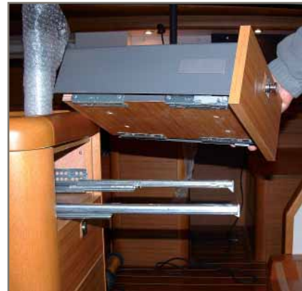
REMOVING THE DRAWER RAILS
