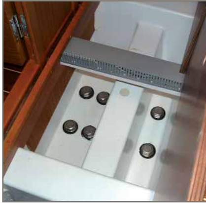
SALOON FLOORBOARD ACCESS TO THE KEEL BOLTS
