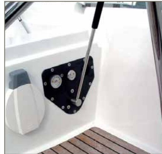
PANEL TO CHECK THE HYDRAULIC BACKSTAYS
