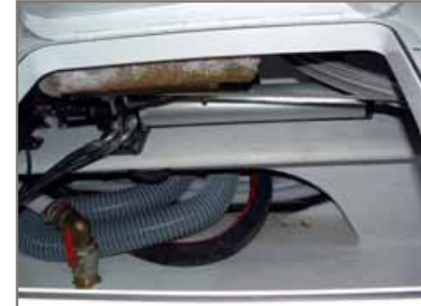
ACCESS TO THE AUTOPILOT IN THE GARAGE
