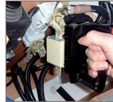
TAKING THE FUSE OUT OF THE THRUSTER - 2
