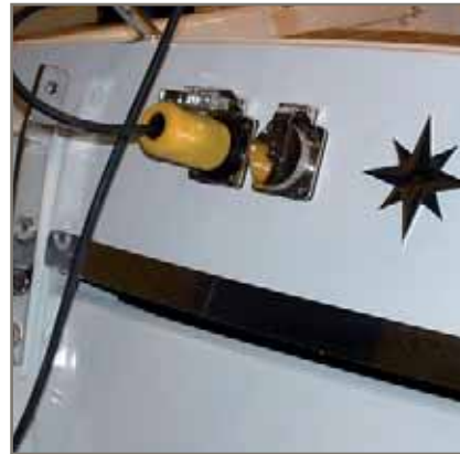
SHORE POWER SOCKETS
